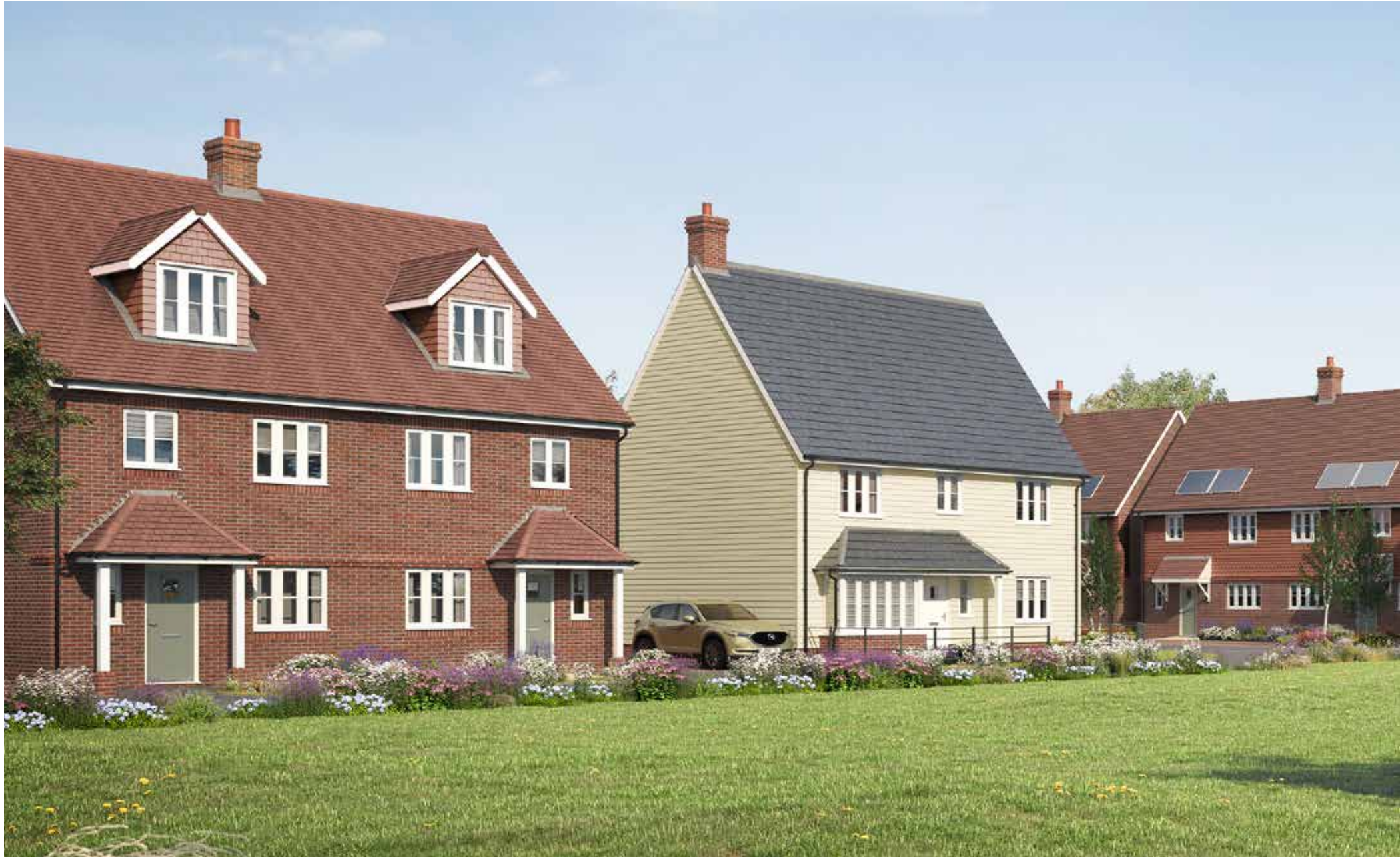
A computer-generated street scene of Mayflower Meadow. The number of PV panels will vary.
